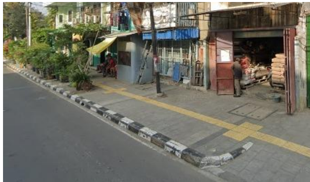
Source: Authors, 2020 Figure 7. Existing condition of pedestrian way within Kota Tua Jakarta, which is not user friendly for disabled people
