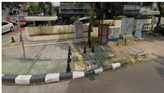
Source: Authors, 2020 Figure 8. Existing condition of pedestrian way within Kota Tua Jakarta, which is many barrier or distraction in the middle of pedestrian way
