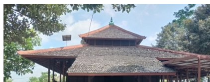
Source: (Author, 2023) Figure 13: Roof of Sunan Drajat's Masjid Makam
