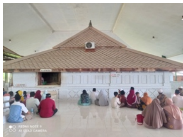
Source: (Author, 2023) Figure 10: Facade of Sunan Drajat's Tomb
