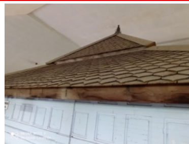
Source: (Author, 2023) Figure 12: Roof of Sunan Drajat's Cungkup
