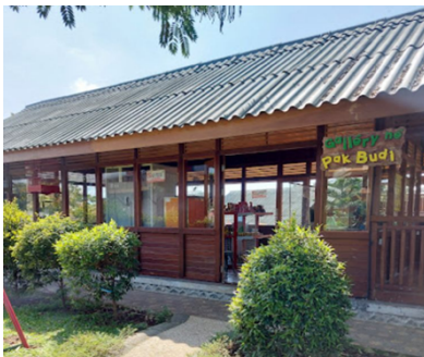
(Source: Personal Documentation, 2024) Figure 6. Canteen Area
