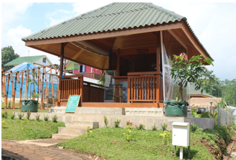
(Source: Personal Documentation, 2024) Figure 9. Gazebo
