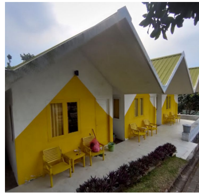
(Source: Personal Documentation, 2024) Figure 10. The repeating pattern of the Cottage
