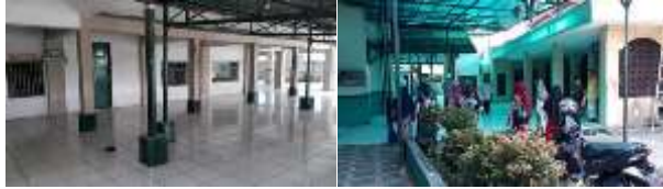
Figure 9. Side hall (left) and Terrace Foundation (right)
