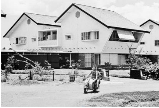
Figure 2. A Scene From 'Tiga Dara' showing Jengki House
