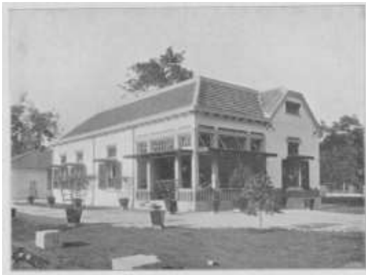
Figure 3: A modern house in Batavia, designed by P.A.J. Moojen Source: Ons Huis in Indie , 1908
