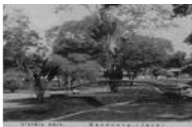
Figure 2: Pieter Park in 1885 (City Hall) Source: (Hariato Kunto, 1984)
