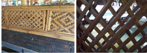
Figure 7: Bamboo Construction with Pelupuh Technique Source: (Personal documentation, 2019)
