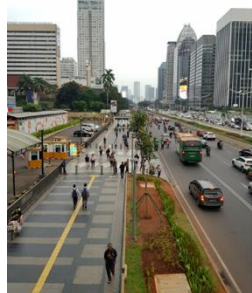
Figure 11: Pedestrian path condition, has 7-8-meter wide, natural stone material, yellow blind pattern for disabled users, and park as separated between pedestrian path and vehicle road. Source: (Author, 2020)
