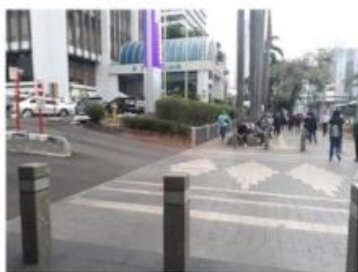
Figure 16: Provided concrete pole with 1-meter height to protect pedestrian from vehicle Source: (Author, 2020)
