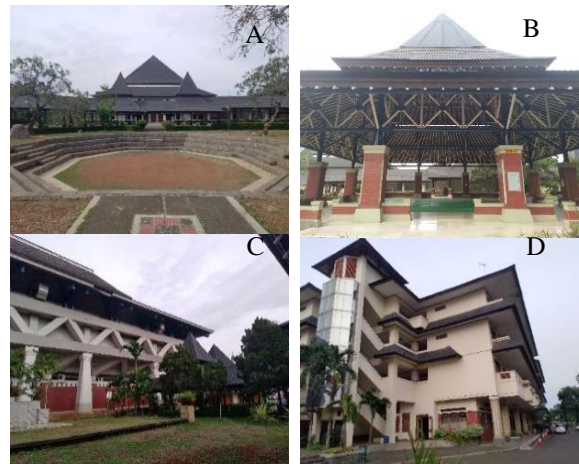
Source: (Personal documentation, 2019) Figure 5: Arena Tanding Terbuka with background of Pondok Serbaguna (A), Pendopo (B), Pondok Gedeh (C), and Pondok Penginapan (D)
