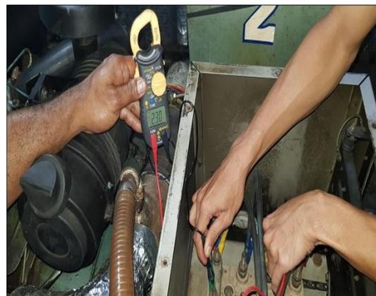
**Fig. 5.** Check the generator output voltage with neutral
