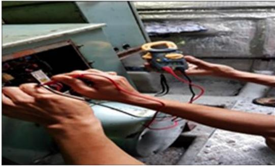
**Fig. 6.** Voltage check on AVR
