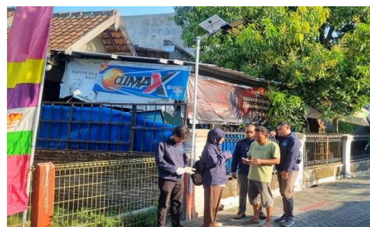
Gambar 5. Uji fungsi remote kontrol PJU panel surya
