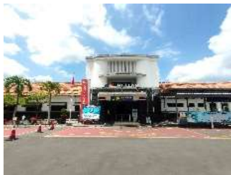
Source: (Antariksa, 2022) Figure 3: Blitar Train Station
