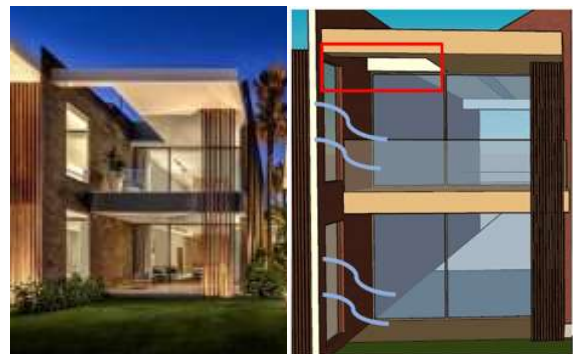
Source: (Author, 2022) Figure 5: Uluwatu House Facade
