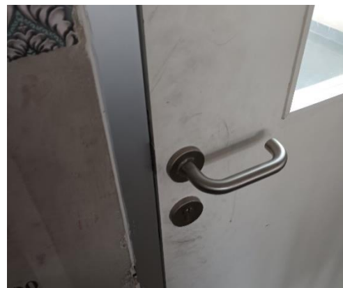
Source: Personal Data, 2023 Figure 5: Classroom door frame and door
