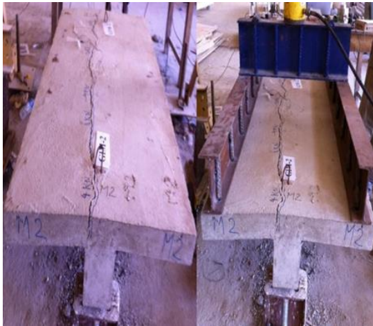
Figure 7. Cracks pattern of specimen GIM-2
