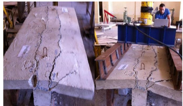
Figure 12. Cracks pattern of specimen GIID-1
