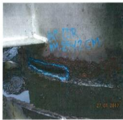
Figure 2. Other hole due to External Corrosion (circular) with dimension 9.8" length and 0.8" width at 12:00 o'clock position also found on flare stack (riser) at connection Ring for guy wire.
