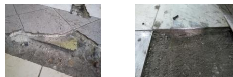
Figure 4.18 the addition of a layer of cement mortar performed
