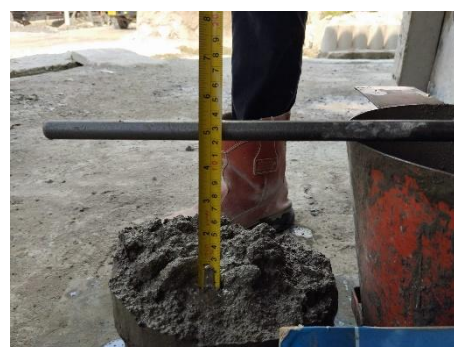
Picture 3. Concrete Slump Test
