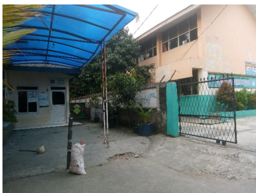
Figure 4. RW 04 office (source: private documentation)
