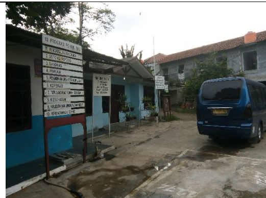
Figure 7. RW 08 office (source: private documentation)
