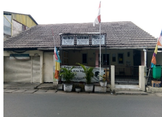
Figure 12. RW 09 office (source: private documentation)
