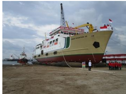
Figure 2. Ship's launching with air bag [18]
