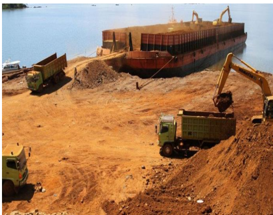
Figure 1. Mining infrastructure work [19]
