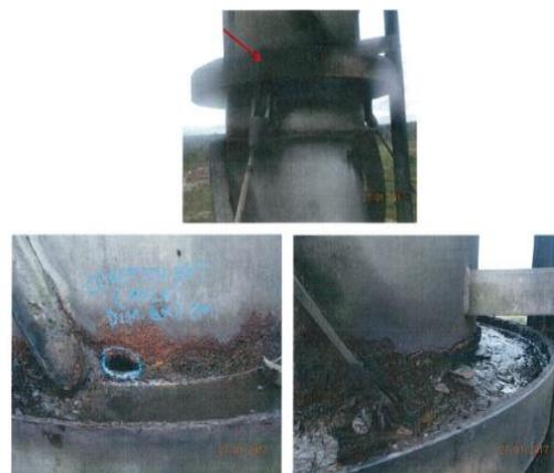
Figure. 1 Hole due to External Corrosion (circular) with dimension 2.4" length and 1.2" width at 18.00 o'clock position on flare stack (riser) of connection Ring area of F-2900A. The nominal thickness of flare stack (riser) is 36" OD x 0.250" thick.
