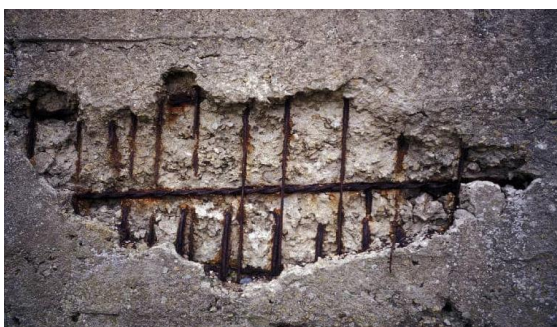
Gambar 2. Spalling Beton [6]
