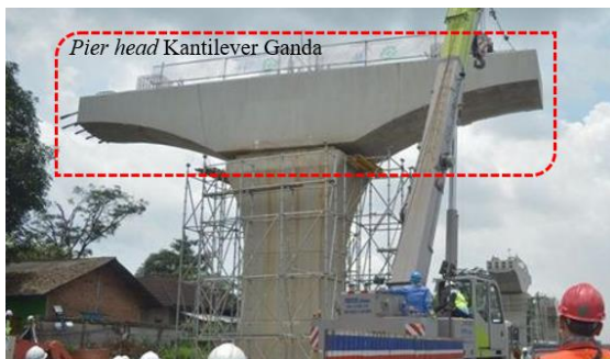
Gambar 1. Contoh Pierhead Kantilever Ganda [8]
