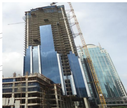
Gambar 4. Facade curtain wall unitized sistim . Sumber : Facade Principales of contruction
