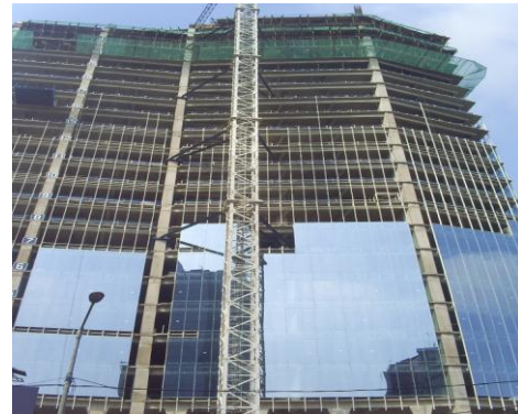
Gambar 3. Sistem stick mullion facade curtain wall. Sumber: Facade Principales of contruction
