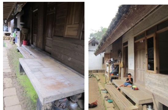
Picture 5. The Facade with New Materials (Source: Private Documentation, 2013)
