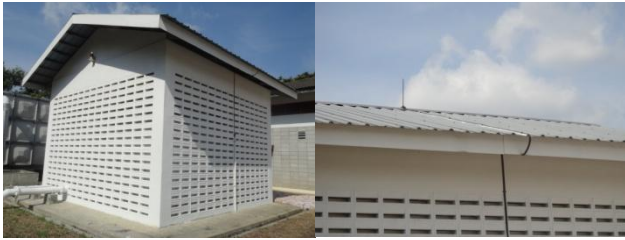
Figure 2. Experimental building with metallic roof Source: Private documentation, 2011
