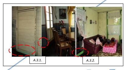
Figure 5: Beams above the floor as the boundaries of spaces found in the Malay traditional Malay dwellings of West Kalimantan
