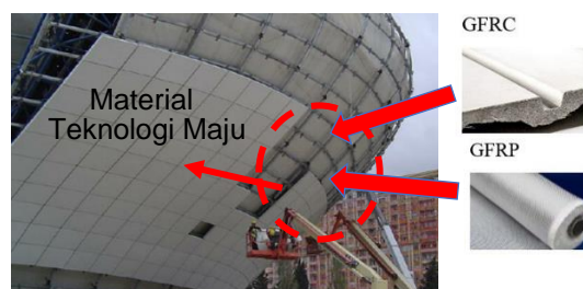
Gambar 16 Proses Pemasangan Material Heydar Aliyev Center. Sumber : https://www.researchgate.net/ , 2022.
