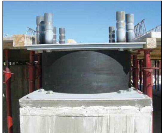
Gambar 11. Base Isolation Sumber : realestate.co.jp (2017)
