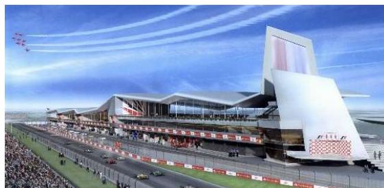
Gambar 8. Pit Building, Sirkuit Silverstone Sumber : Kumar (2015)
