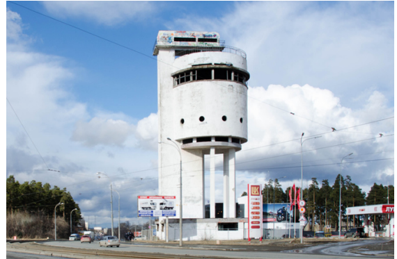
Gambar 4: Old Water Tower
