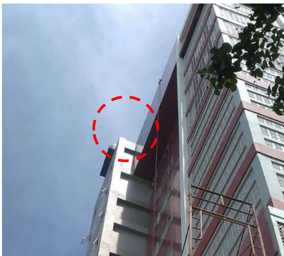
FIGURE 3. Making processing and final results of realized installation design with 2 Cyclone Configuration.
