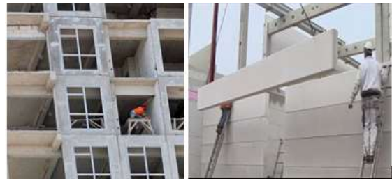
Gambar 4.1.6 Penerapan autoclaved aerated concrete Sumber: (Analisa Pribadi, 2020)
