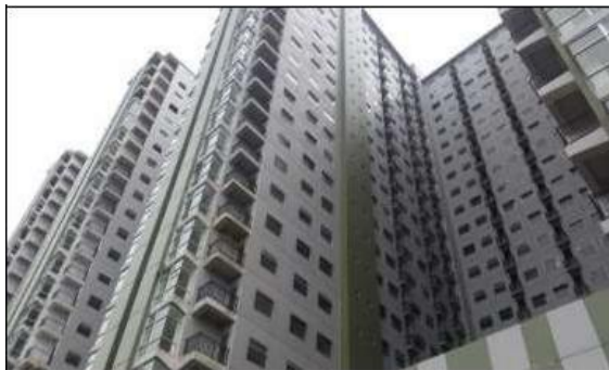
Gambar 1. Gedung Apartemen Grand Asia Afrika Residence.
