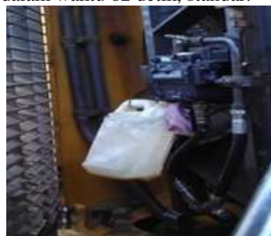
Gambar 3.70. Testing internal leak
