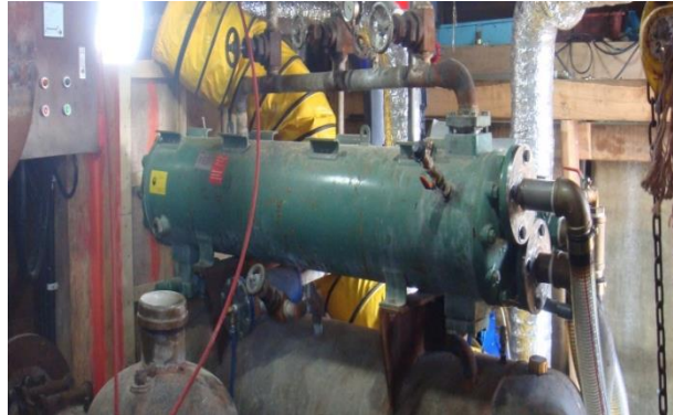
Gambar 5. Kondensator Bitzer
