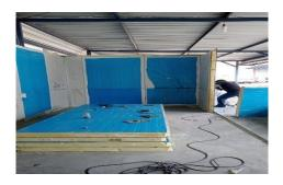
Gambar 3. Pemasangan dinding coldstorage
